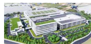
Electrification Innovation Center (Anjo Plant)
