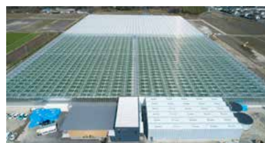
Rendering of a large-scale greenhouse at AgriD Location: Inabe City, Mie Prefecture; Scale: 4ha (cultivation area)
