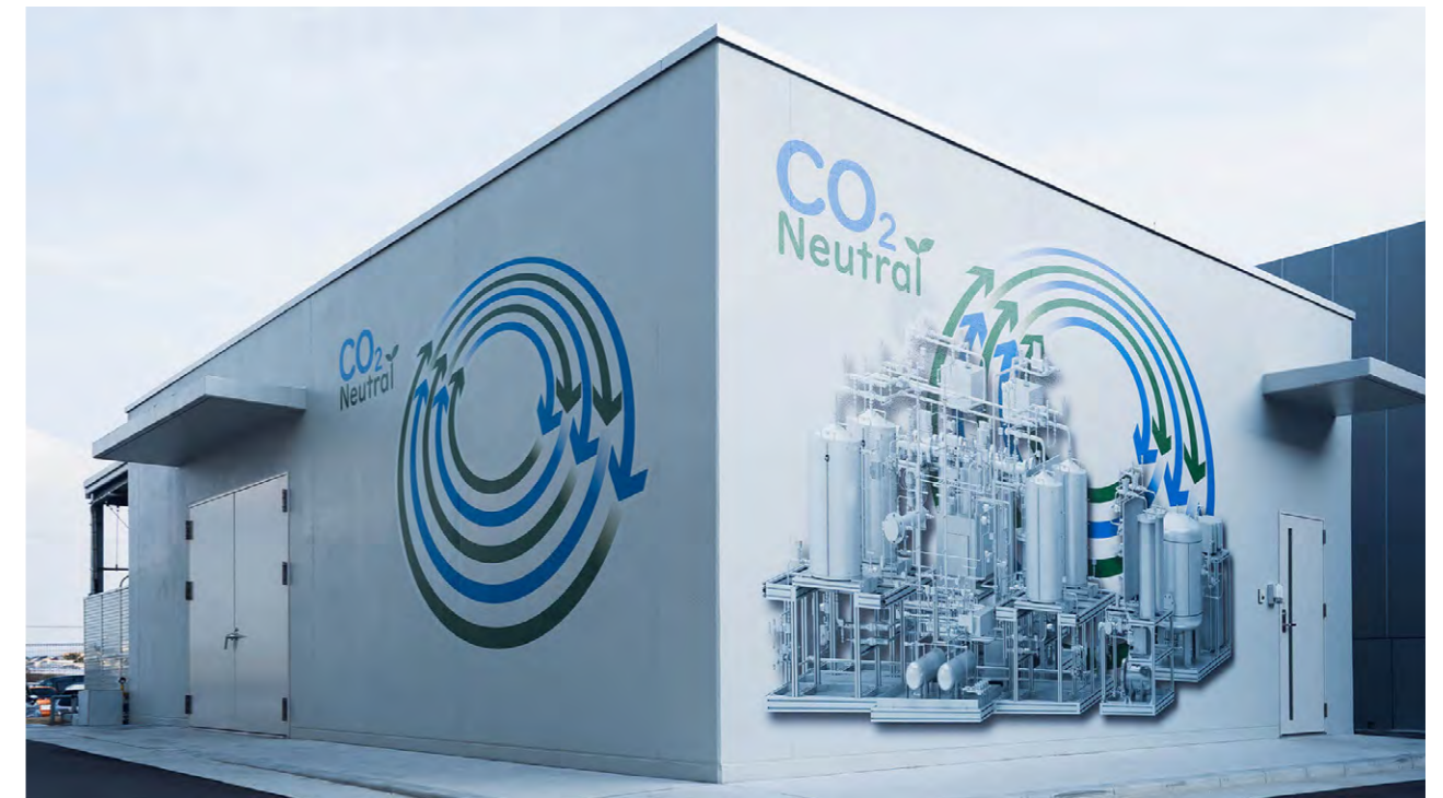
The CO 2 Circulation Plant was built adjacent to the Anjo Plant in Aichi Prefecture. The plant was completed through joint technological development with Toyota Central R&D Labs., Inc.
