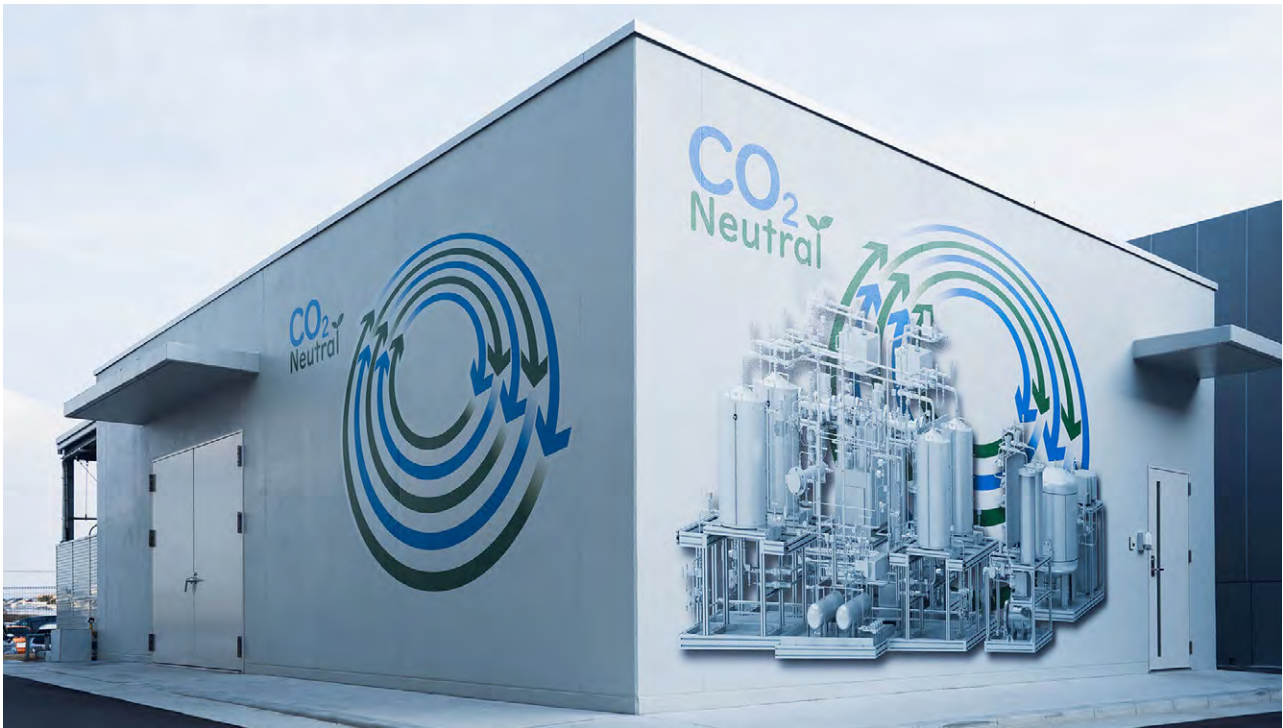
The CO 2 Circulation Plant was built adjacent to the Anjo Plant in Aichi Prefecture. The plant was completed through joint technological development with Toyota Central R&D Labs., Inc.
