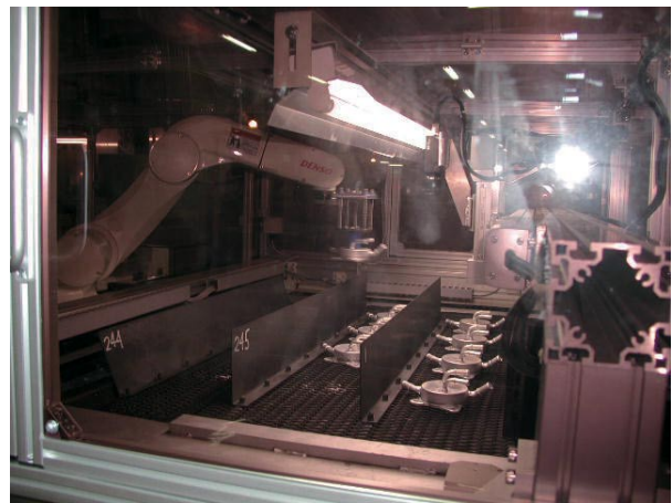
Fig. 14 Photo of the end of the furnace
