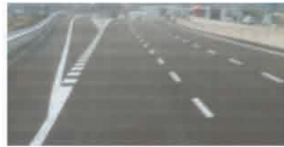
Fig. 5 Lane Mark Shapes Marking Expressway Branch off Point
