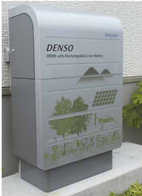
Fig. 4 Exterior of Li-ion Battery System
