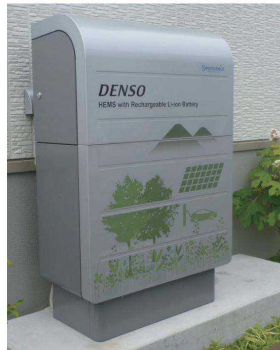
Fig. 1 External appearance of Li ion battery system for HEMS
